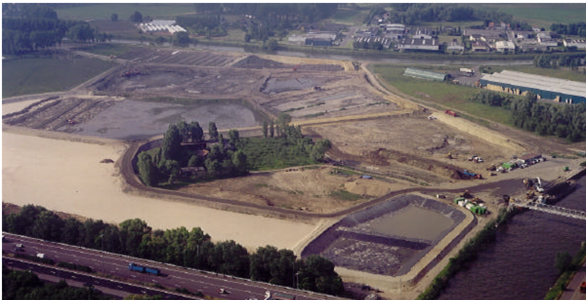
Figure 5: Sludge Treatment Centre 'Fasiver'
