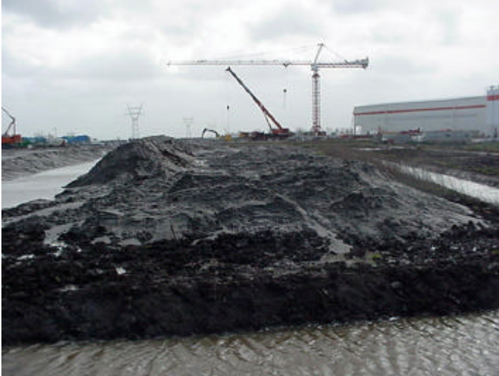
Figure 3: Storage of excavated soil
