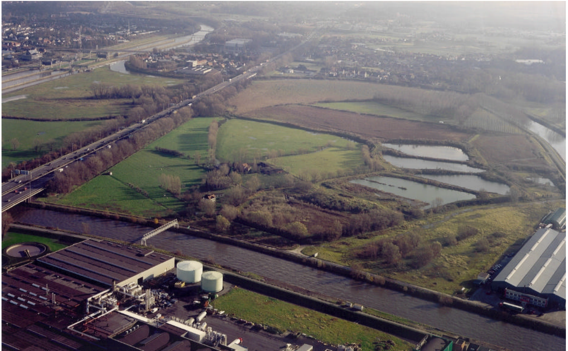
Figure 2: Air view of 'Fasiver'-site
