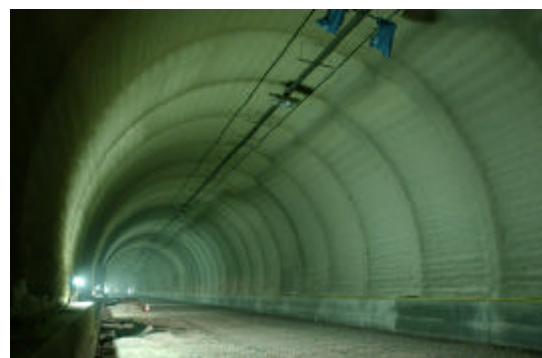
Figure 5: Insight of the Westerscheldetunnel
