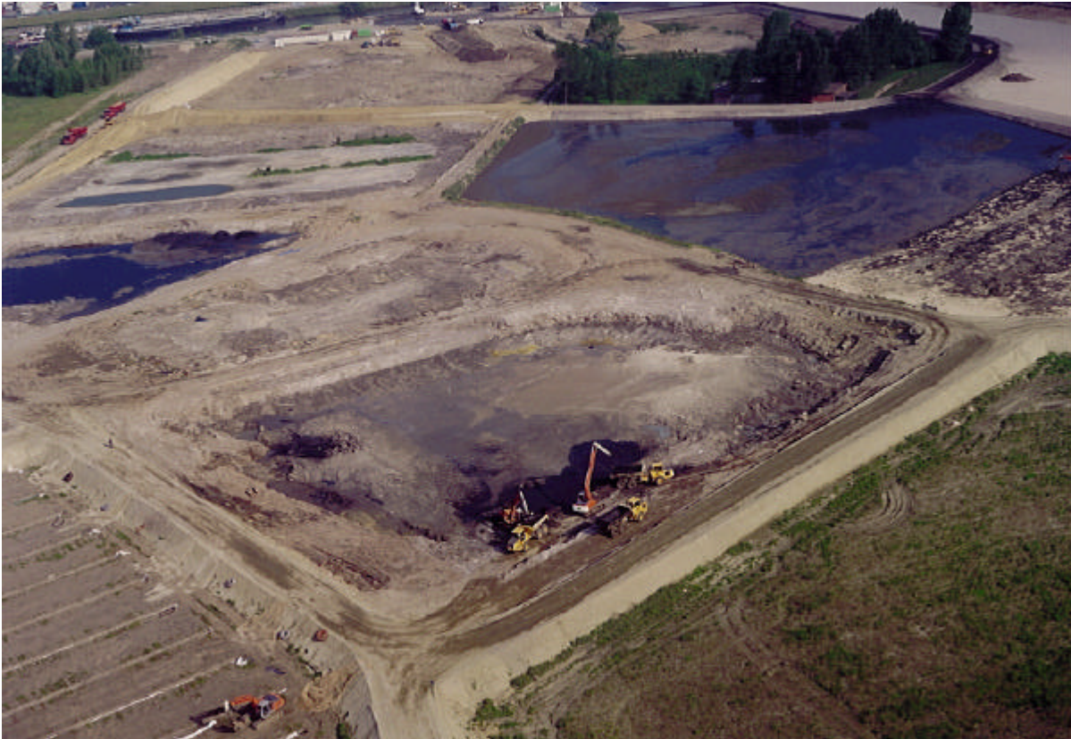
Figure 4: Overview of the stabilisation of the different basins
