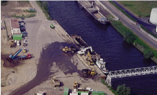
Figure 6: Quay wall at 'Fasiver'-site
