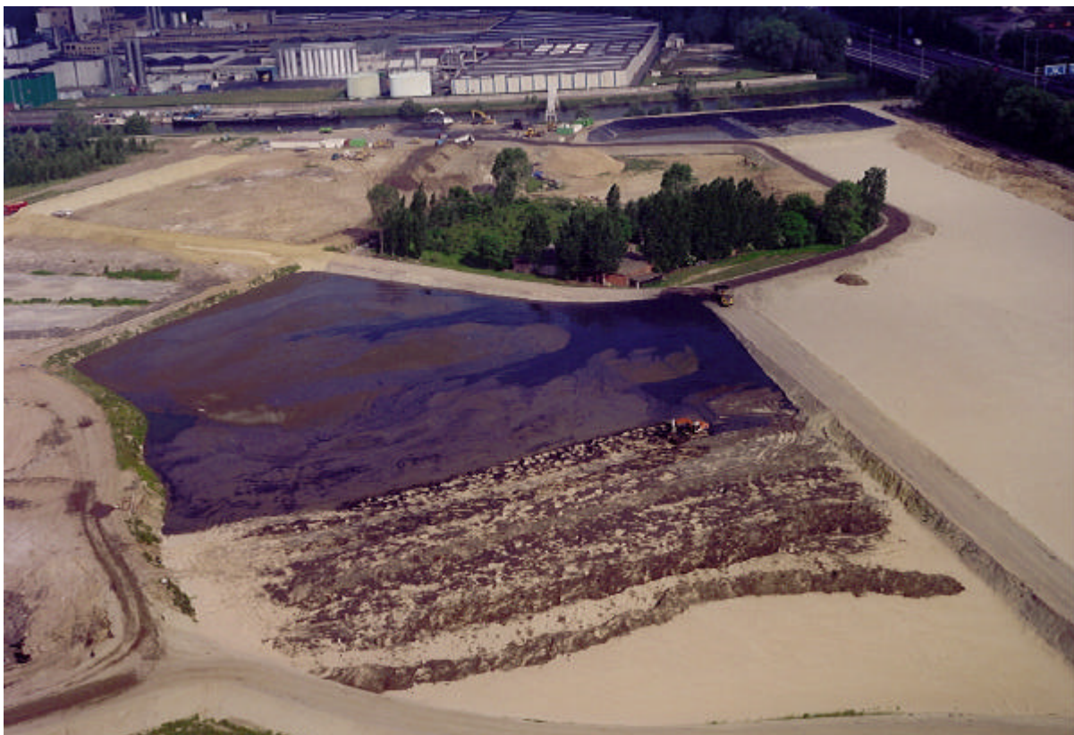
Figure 8: Accelerated natural dewatering of dredged material
