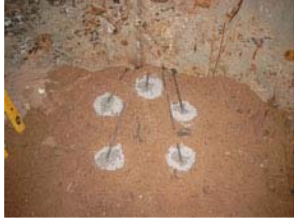
Fig. 9: Installation of the probes inside the pilot column
