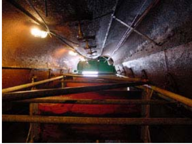
Fig. 4: Space between the columns (gap)
