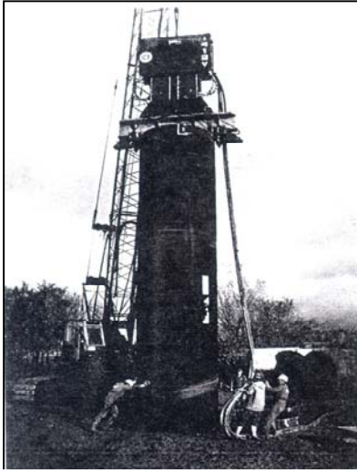
Fig. 3: Ramming of the columns
