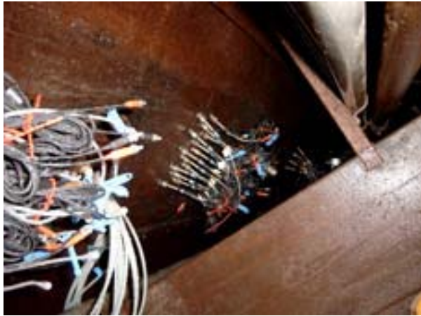
Fig. 8: Installation of the probes outside the pilot column
